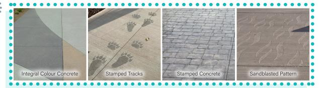
Figure 15: Examples of different concrete surface treatments
