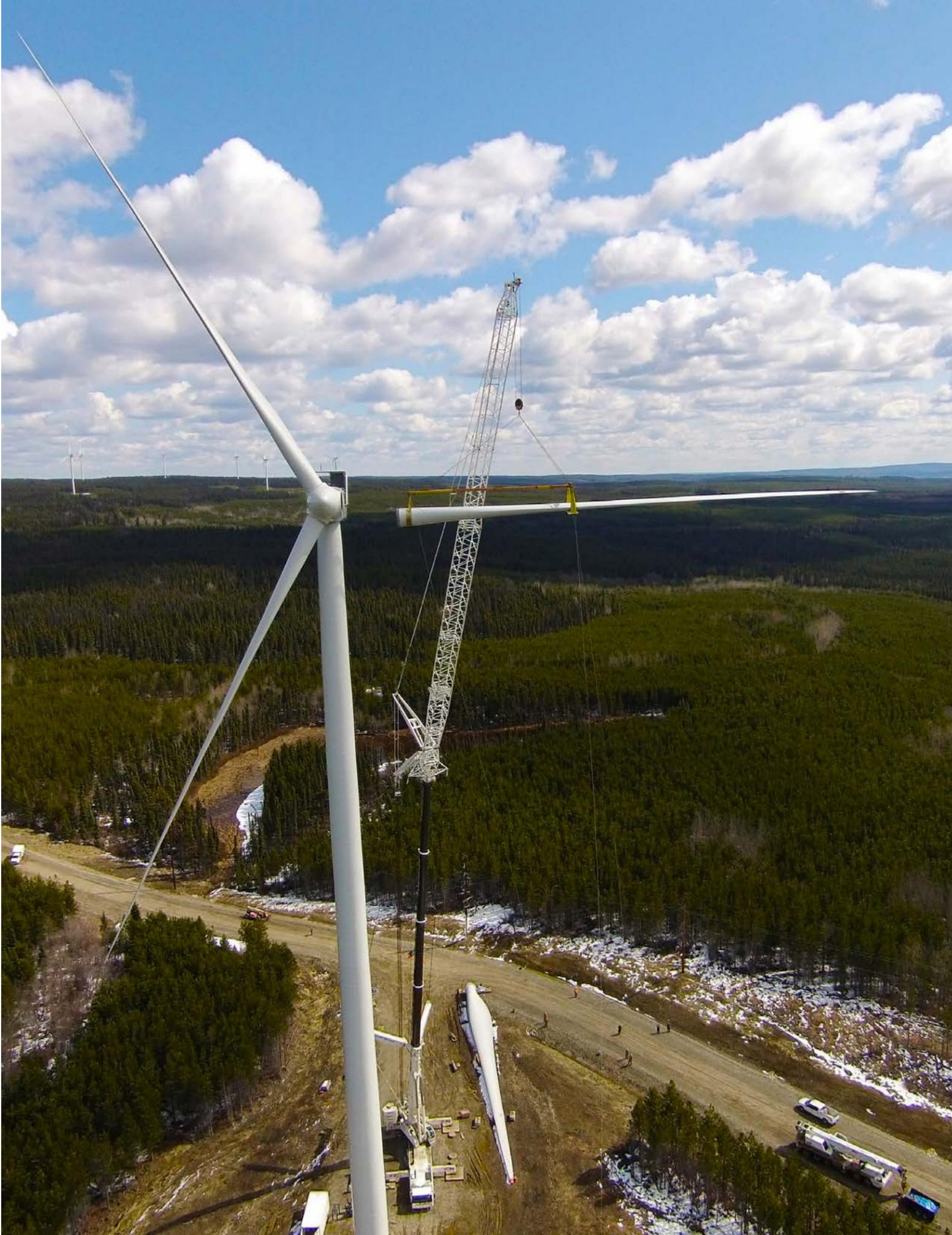
An aerial photograph showing a large white wind turbine under construction. A tall lattice crane is positioned next to the tower, with a long white blade being hoisted into place. The surrounding landscape is a mix of green forest and cleared construction areas with dirt roads. In the background, other wind turbines are visible on a ridge under a blue sky with scattered white clouds.
